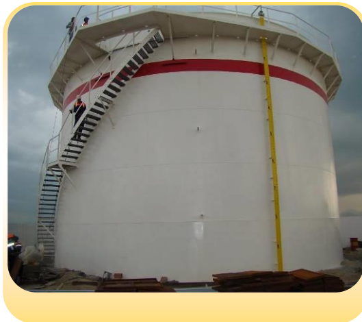
2007: Manufacturing and installation of a water tank 2000 m 3 (Ø16000-H=10000) in Rades – BI/SNDP
