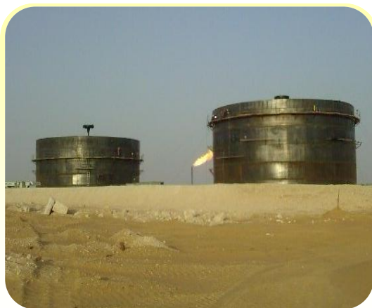
2008: Mounting 02 petroleum tanks 5000m 3 IN DESERT – BI /PIONNER
